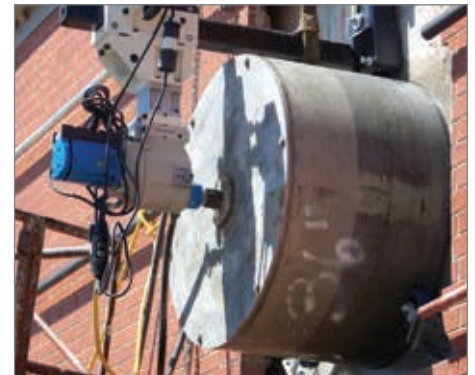
TS-605 drilling with a 36" bit at a water treatment plant
