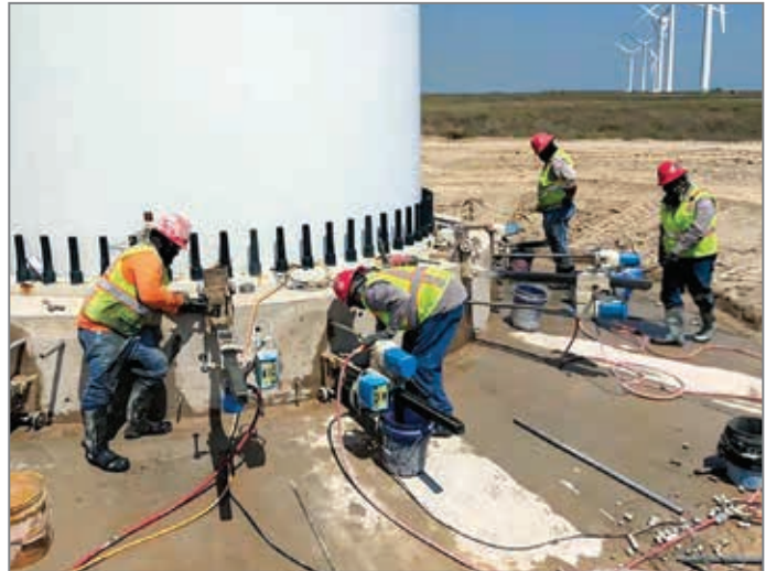
Coring operators running multiple drills at once!
