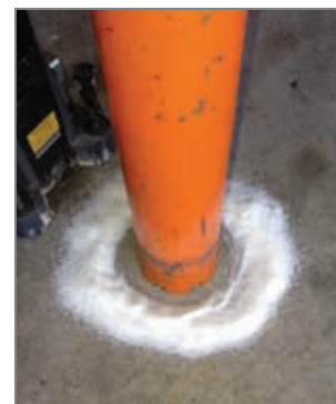
By sprinkling gel around the bit before drilling the water and mess are contained in a small area.
