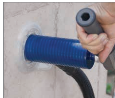
By sprinkling gel around the bit before drilling the water and mess are contained in a small area.
