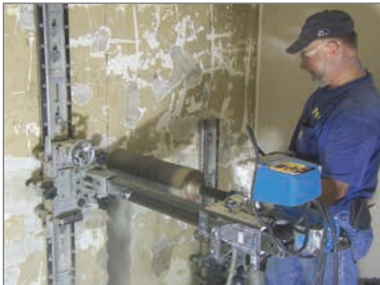
Stitch drill used to drill a series of holes shown with Auto-feed
